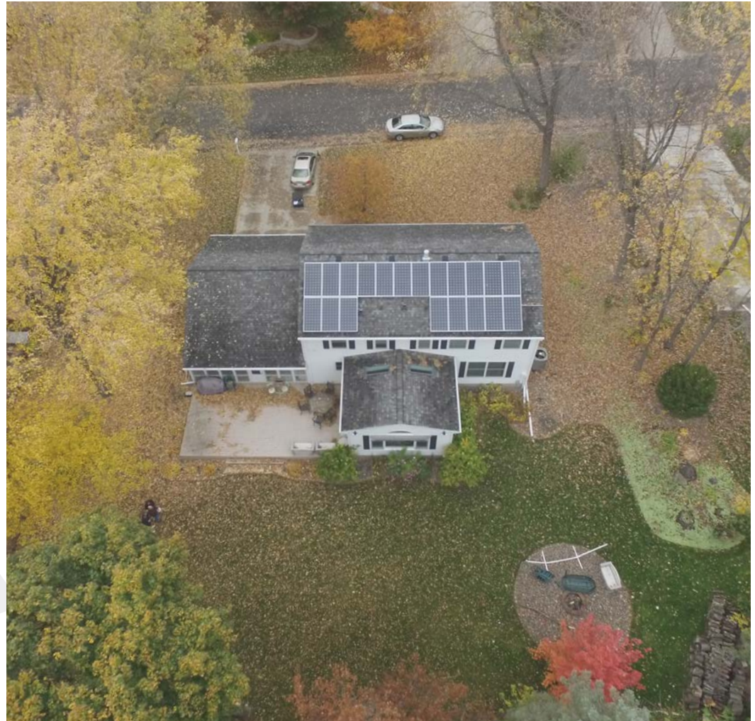
Residential solar panels, photo by Jeff Stuhr, courtesy MPCA
