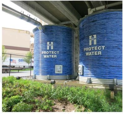
Target Field Station includes a variety of features, including these cisterns and bio swale that capture and filter approximately three million gallons of rainwater and snow annually.
